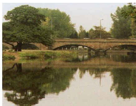
5.0.7 County Bridge over River Dove
